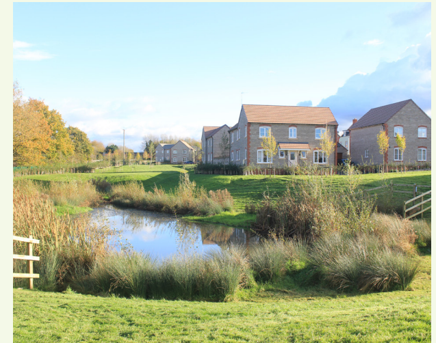
SuDS designed as a natural pond with accessible, split level banks, Ridgeway Farm, Swindon
