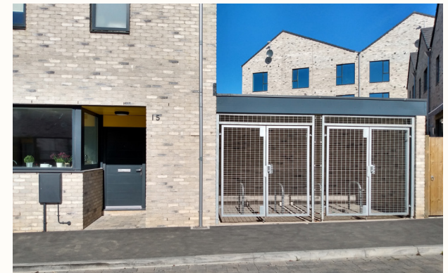
Communal cycle store integrated with end terrace, Bristol
