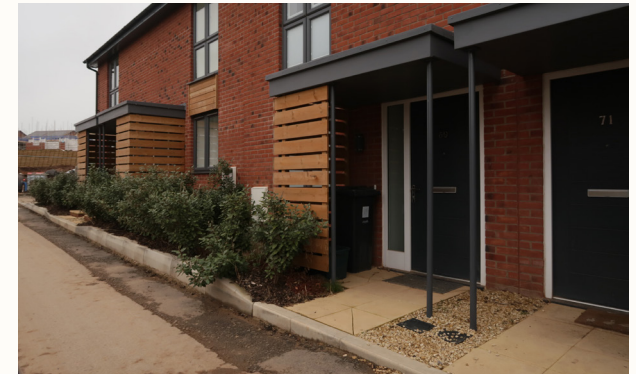
Bin store integrated with terraced frontage, Bristol
