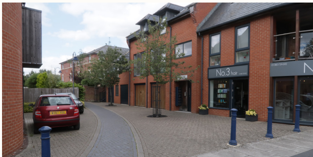
Attached built form and mews, Snuff Street, Devizes
