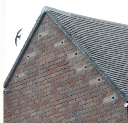
'Universal bricks' integrated within the building's fabric
